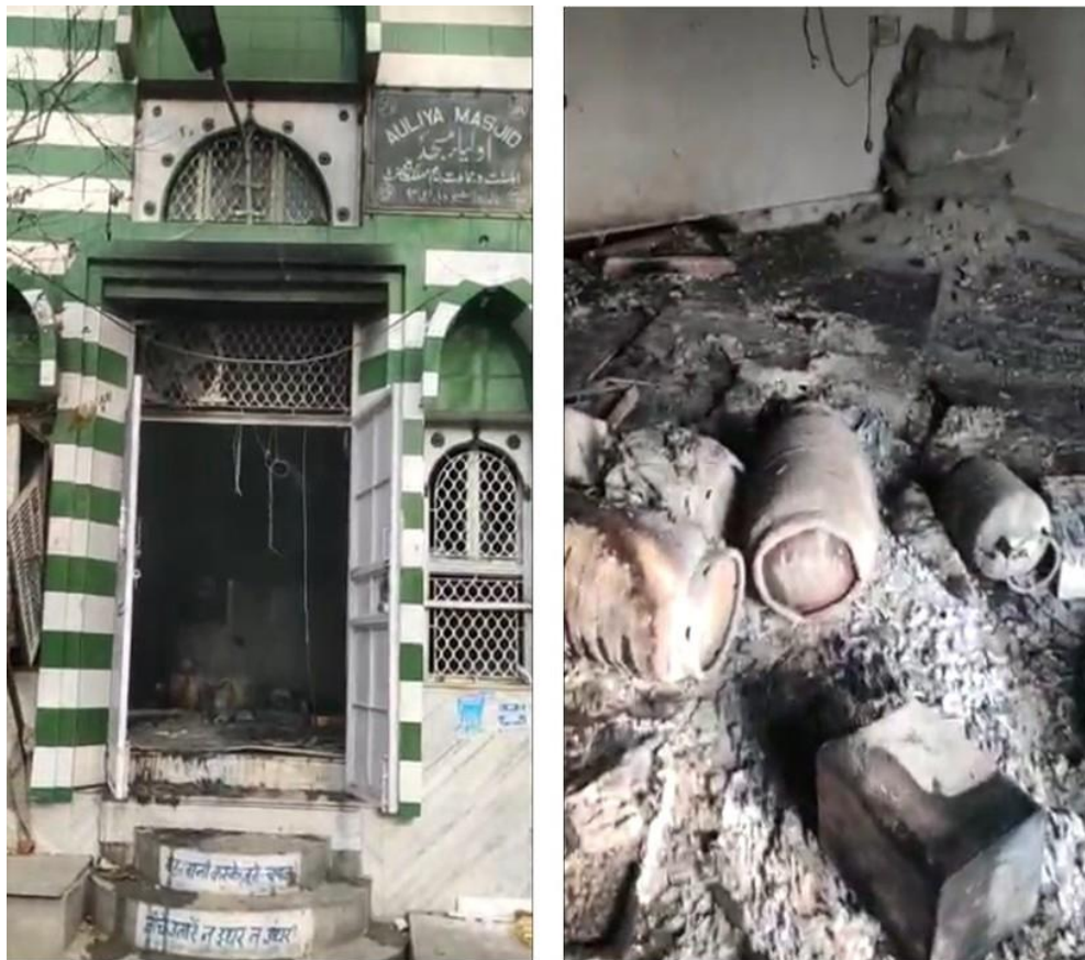
Figure 20: The destroyed Aulia Masjid, Phase 7, Main nullah road, Shiv Vihar.
